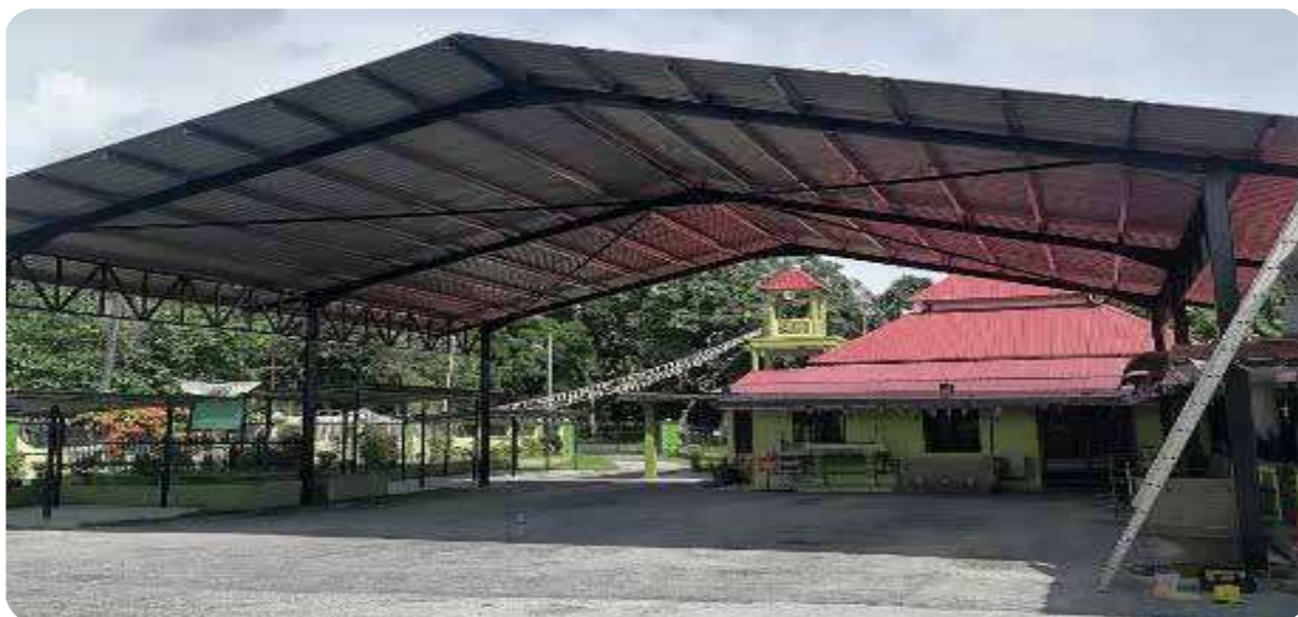
Mild steel roofing structure constructed as part of the mosque development at Masjid Kariah Masjid Tanah Chembong, Negeri Sembilan.
